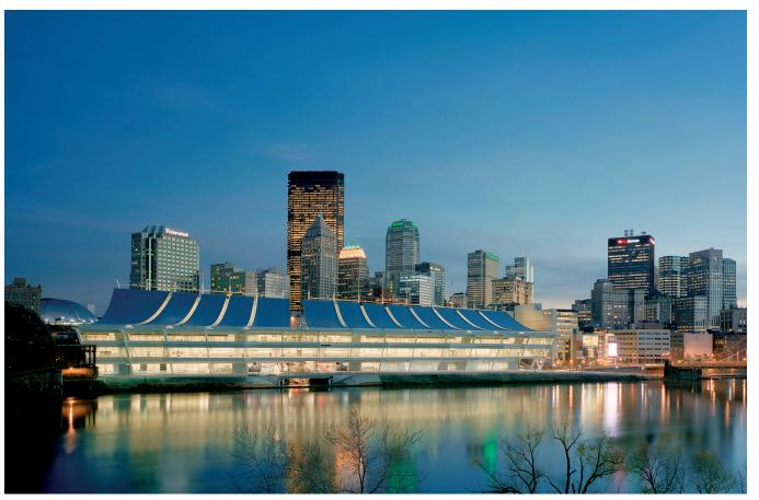
The suspension roof of this 134,700-square-meter (1.45 million-square-foot) convention center integrates into a single sweeping gesture the contextual, environmental, structural, and programmatic requirements of the project. Its iconic design takes inspiration from the historic suspension bridges that span the Allegheny River
